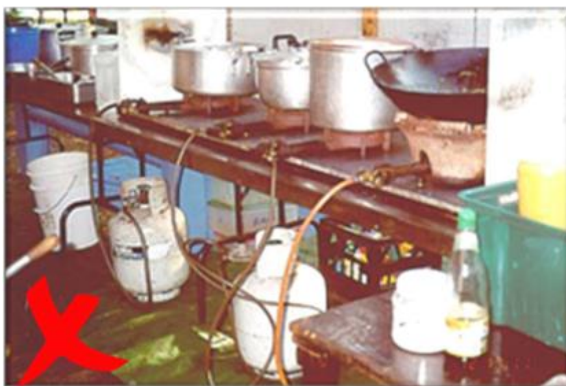
Figure 12. Example of non-compliant gas set up
