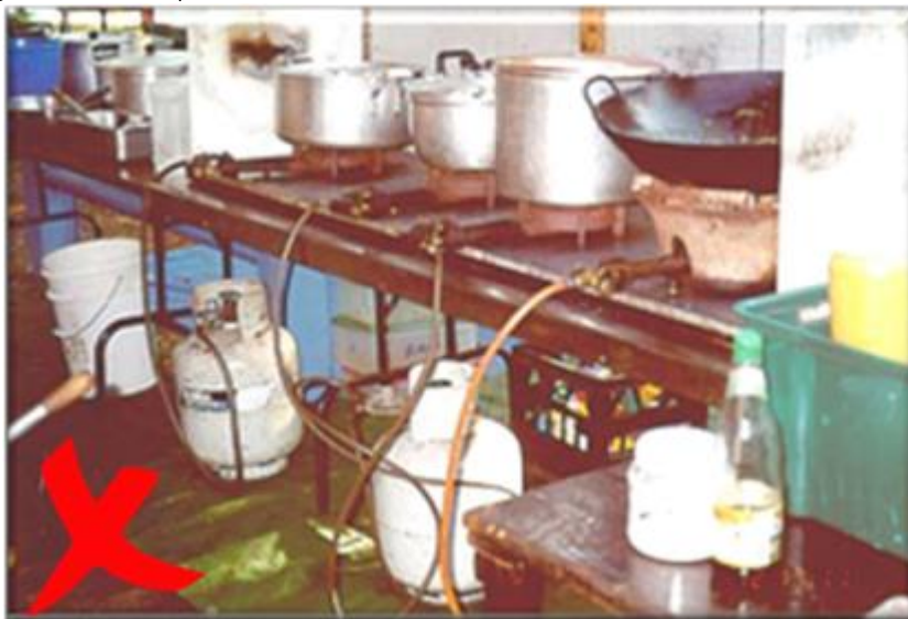
Figure 12. Example of non-compliant gas set up
