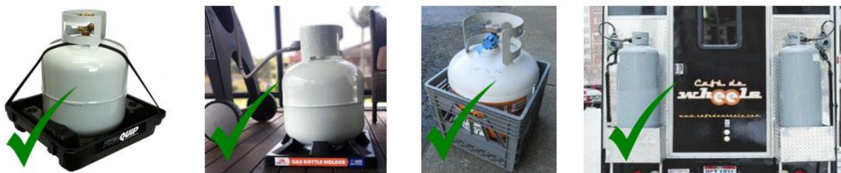
Figure 7. Examples of suitable gas bottle storage
